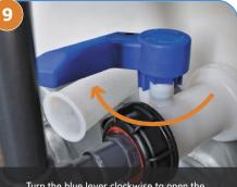
Turn the blue lever clockwise to open the valve at the bottom of the unit.
