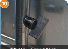
Fit Grab Tap to test outlet on main pipe. Take a sample of condensate once a week and test. (see over for details)
