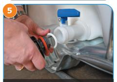
Attach the long outlet pipe to the outlet of the unit by screwing the black ring onto the thread. Ensure that the pipe is fitted with a white sealing ring.
