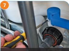
Unlock the valve lever by loosening the screw below the blue lever arm.
